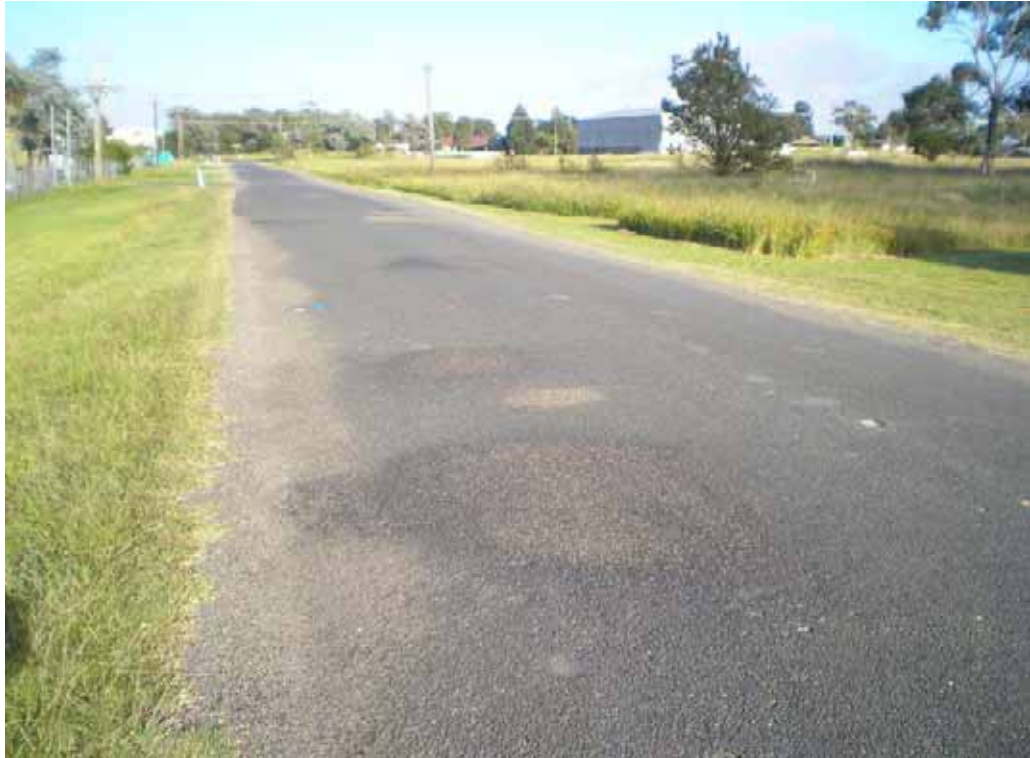
PHOTO 13: Repaired sections
