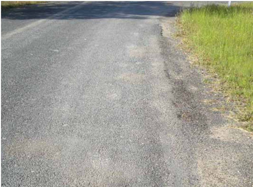
PHOTO 34: Repaired/widened shoulder
