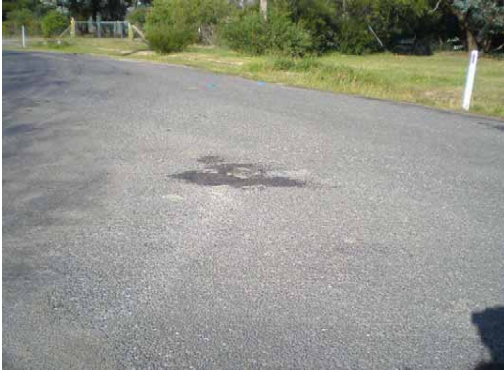
PHOTO 29: Series of pothole repairs
