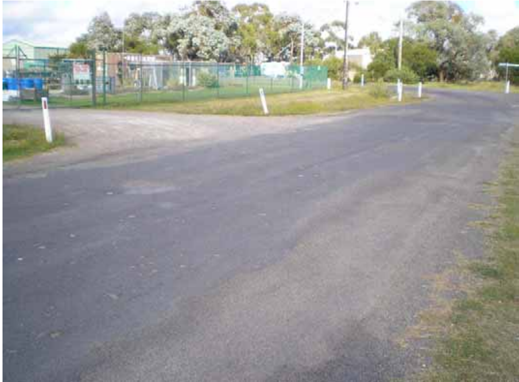
PHOTO 23: Shoulder repair/widening, loss of seal, repaired sections
