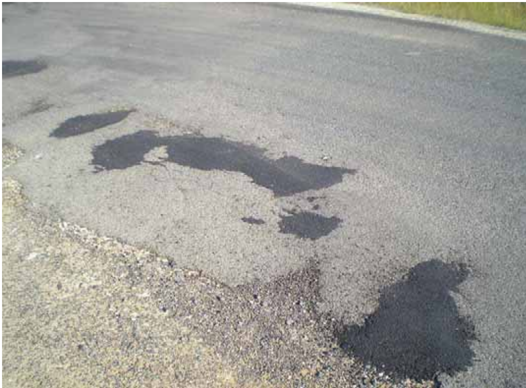
PHOTO 56: Pothole repairs
