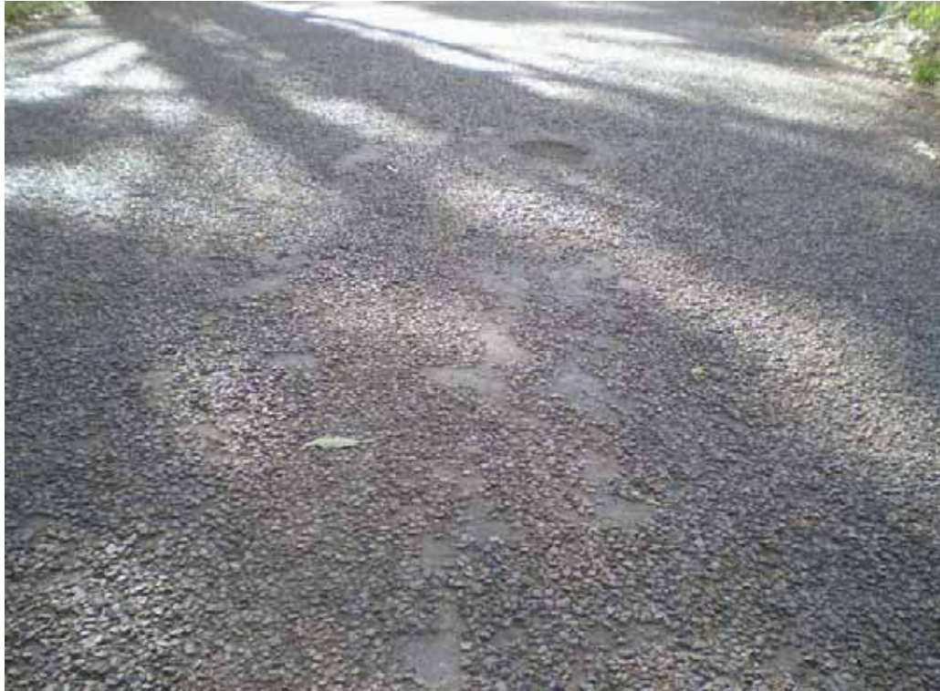
PHOTO 89: Stripped aggregate, repaired pothole
