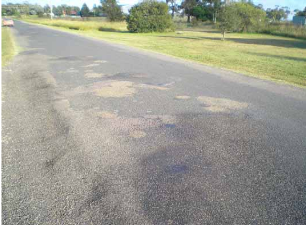
PHOTO 11: Repaired sections/potholes
