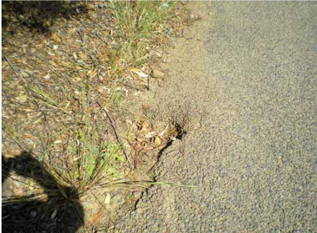
PHOTO 105: Pavement edge repairs and erosion
