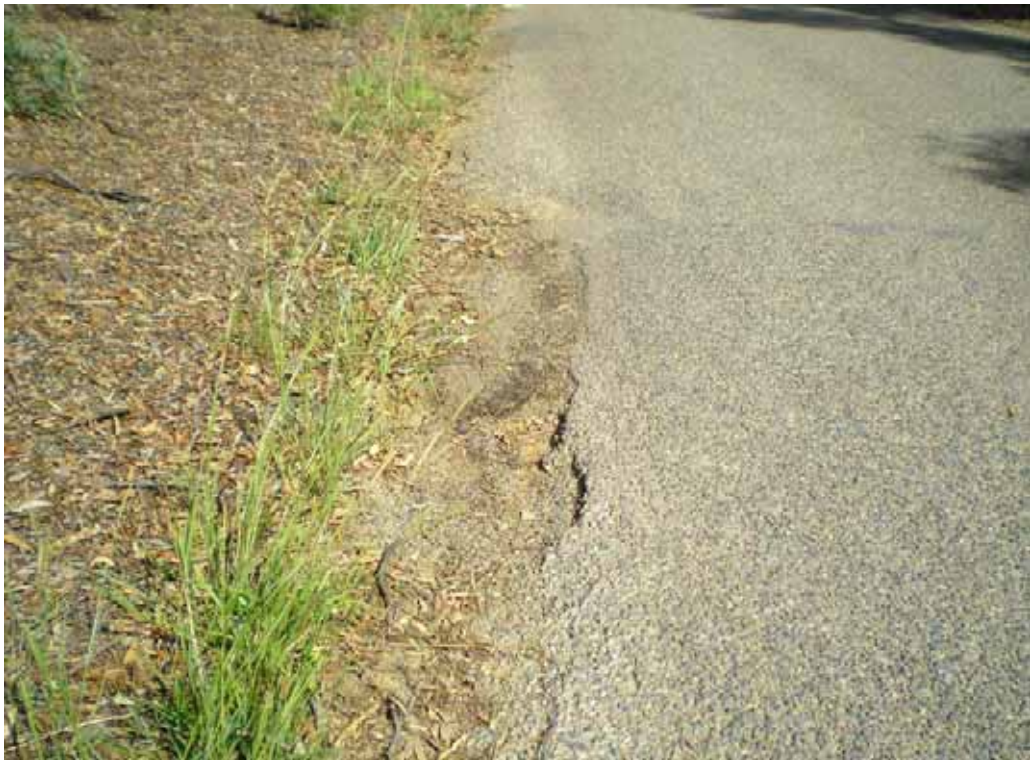
PHOTO 106: Pavement edge repairs and erosion
