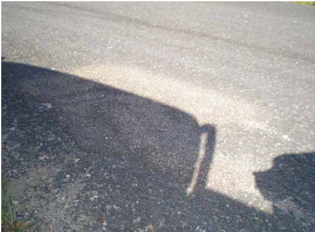
PHOTO 74: Repaired pothole
