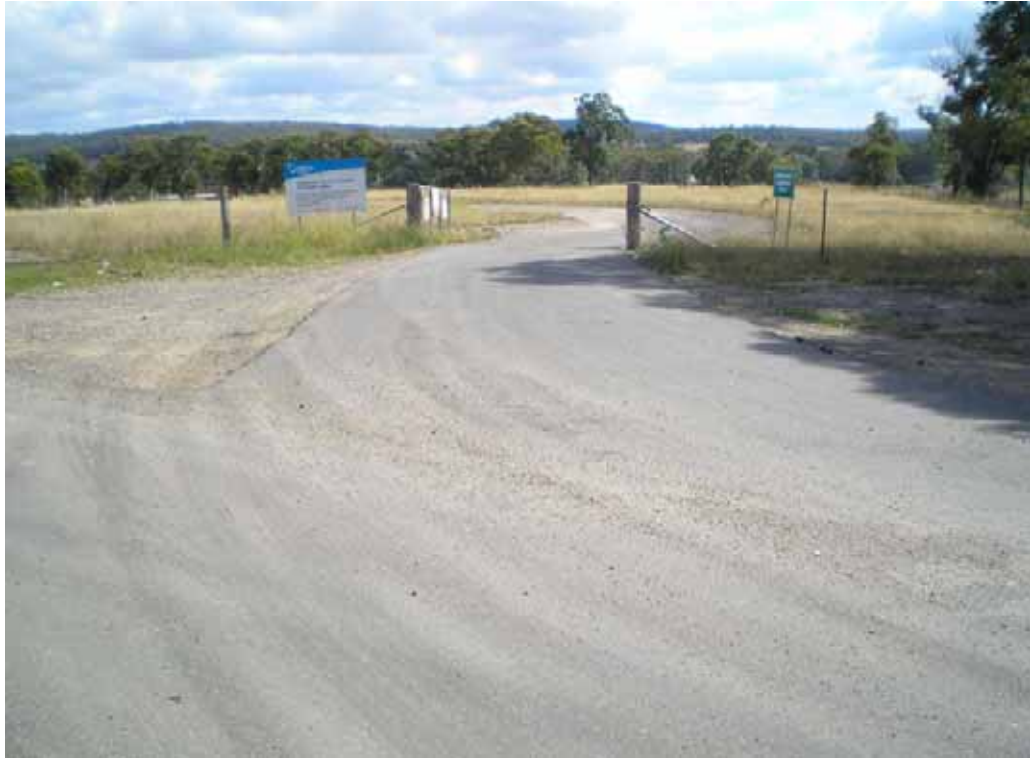
PHOTO 111: New seal at Orica gate
