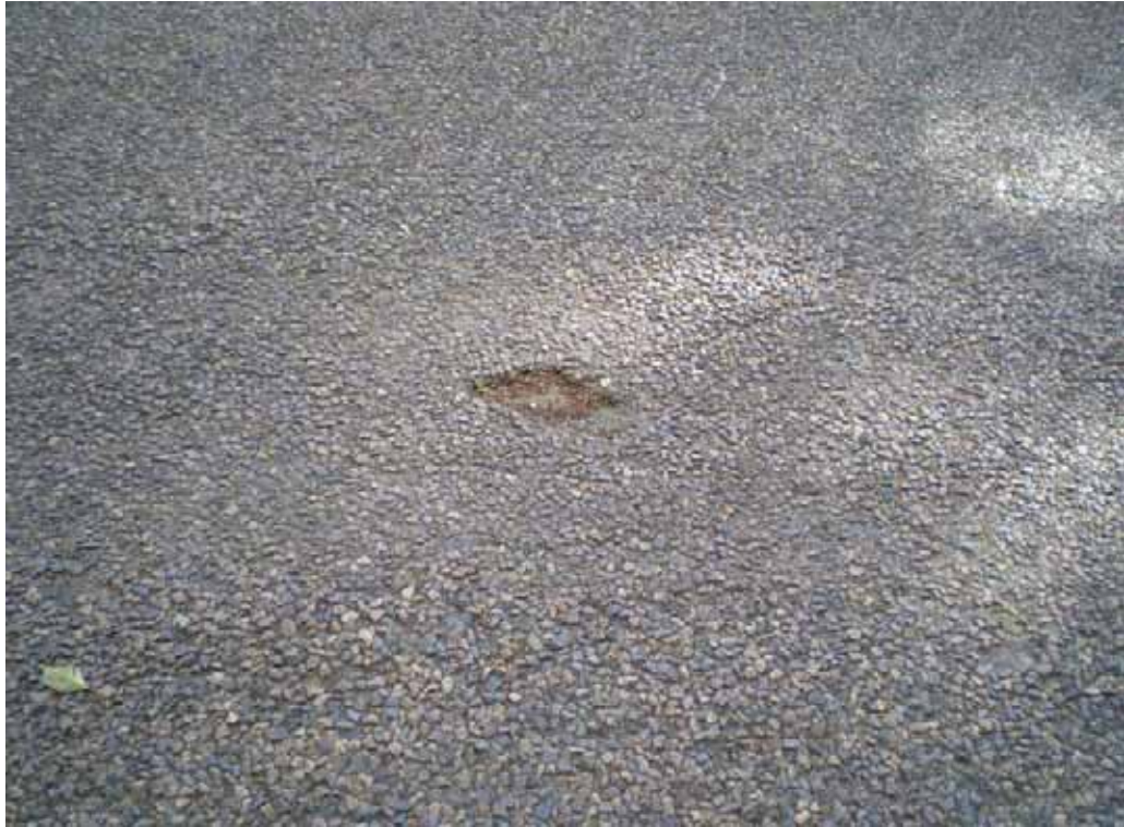
PHOTO 101: Small pothole
