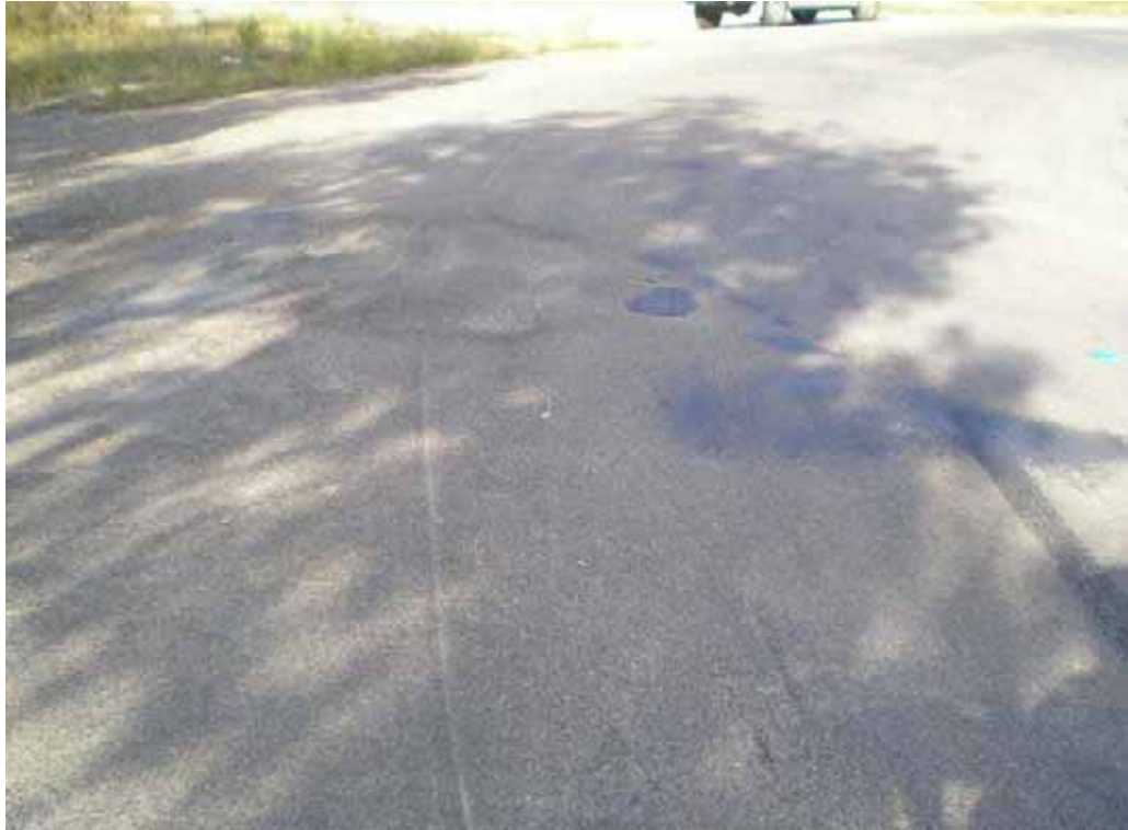
PHOTO 39: Repaired potholes, gauging in asphalt
