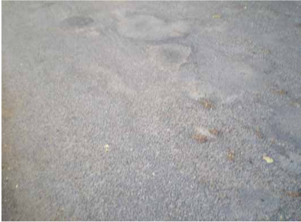
PHOTO 87: Repaired potholes
