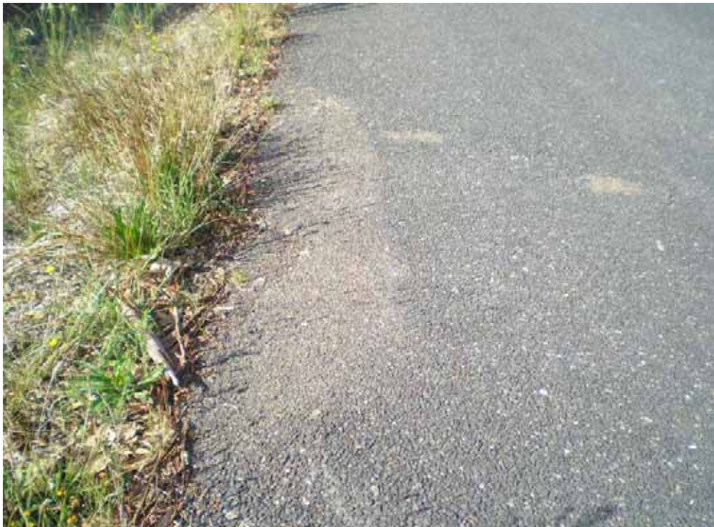
PHOTO 68: Repair in pavement edge
