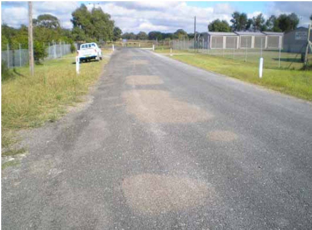
PHOTO 50: Repaired sections
