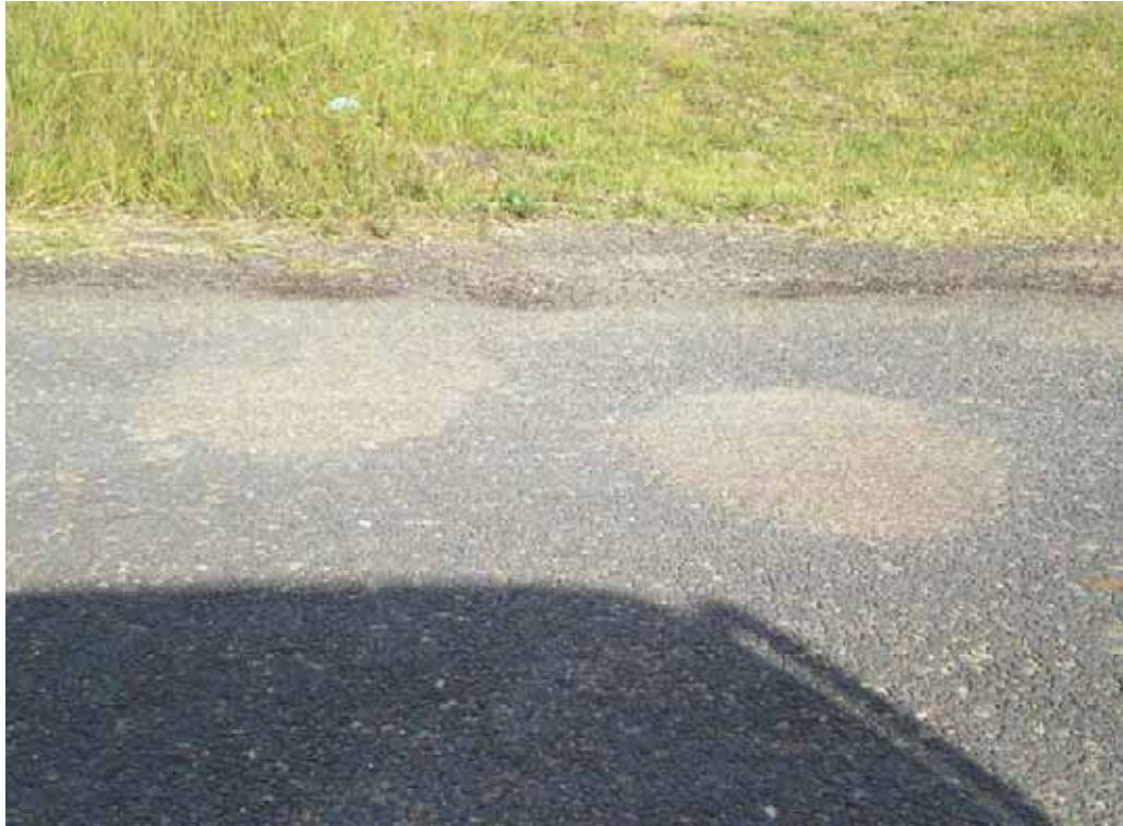
PHOTO 33: Repaired potholes
