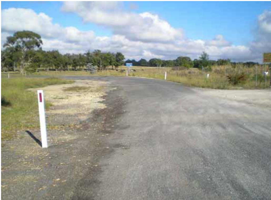
PHOTO 52: Concrete batch plant entrance
