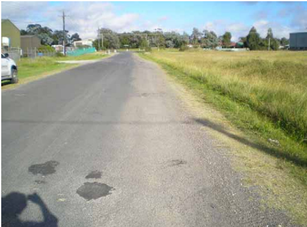
PHOTO 16: Shoulder widened/repaired
