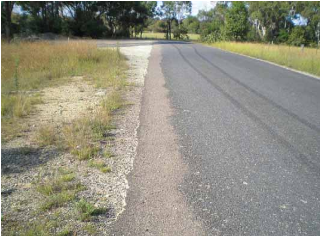
PHOTO 78: Shoulder widening/repair
