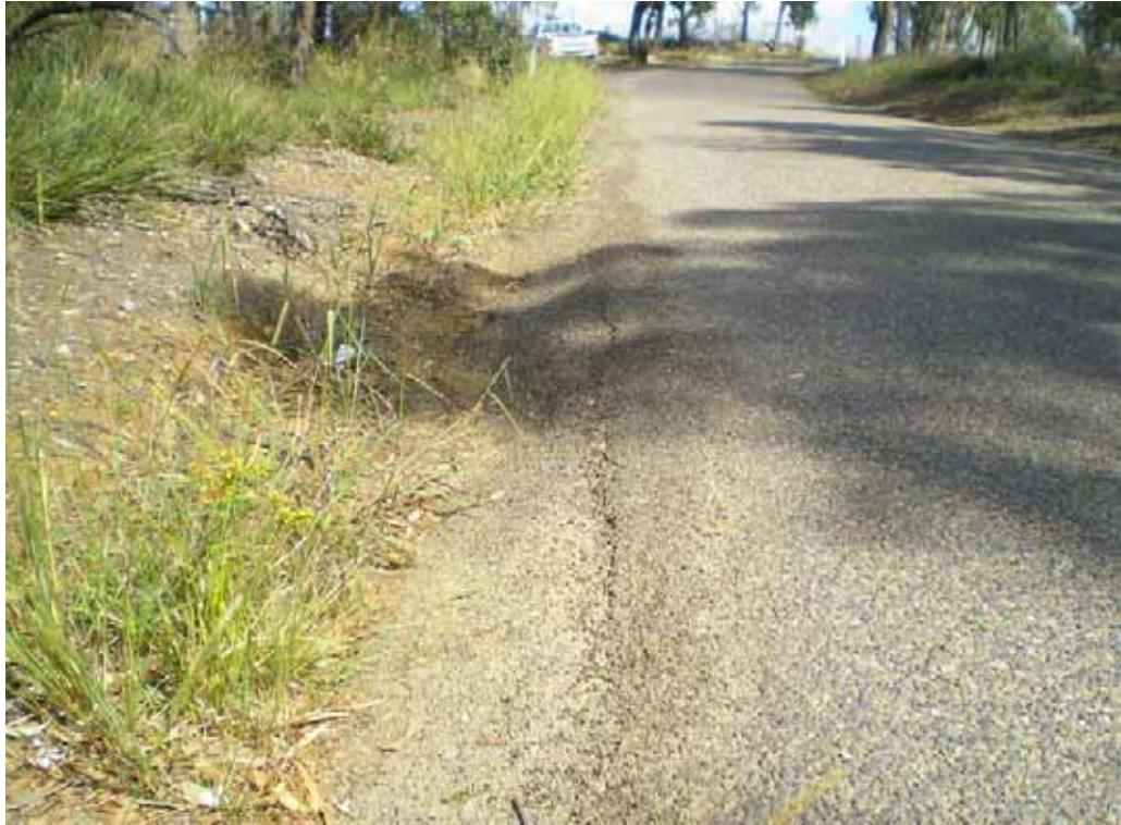
PHOTO 109: Pavement edge repairs
