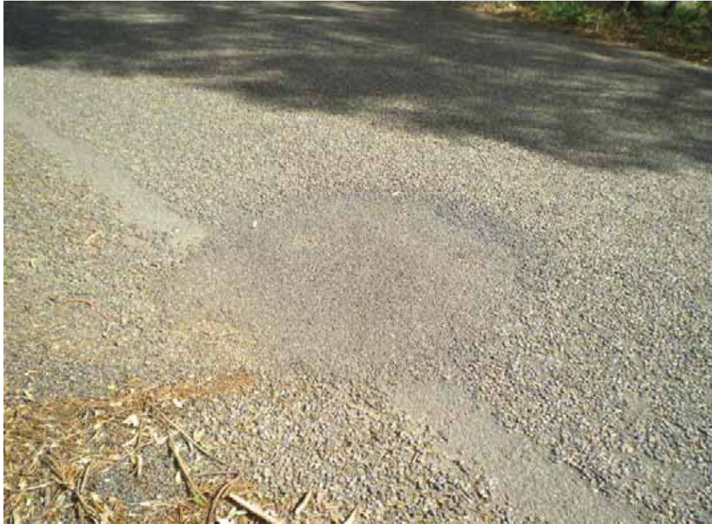
PHOTO 97: Repaired pothole, shoulder repair/widening
