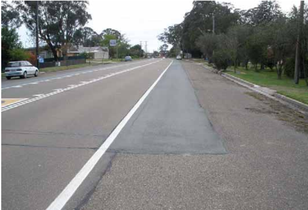
Photo 19 – Opposite No 36 George St. Resealed shoulder (east).
