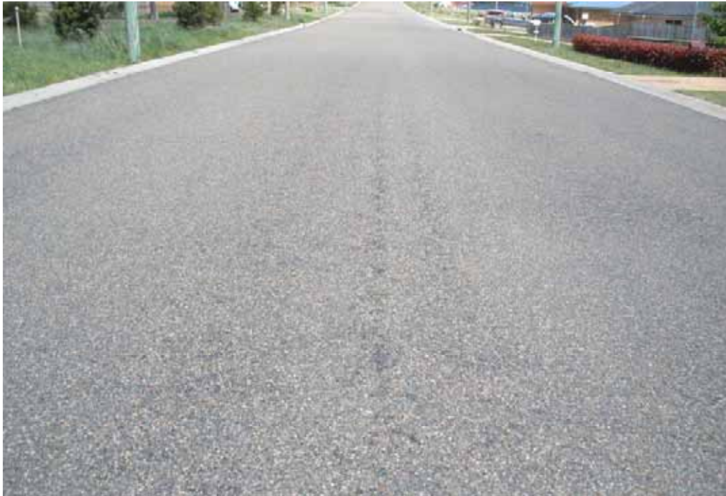
Photo 91 – Opposite No 29 Stoney Creek Rd. Aggregate loss near centreline and slight rutting.
