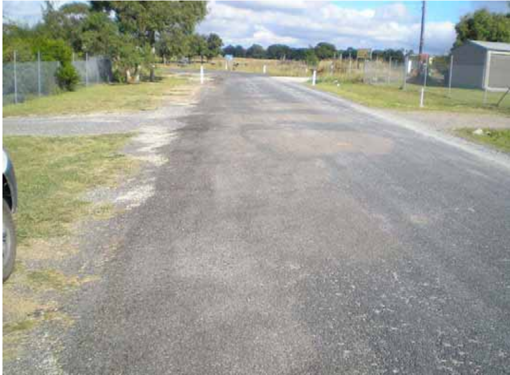
PHOTO 51: Shoulder and pavement repairs, settlement at shoulder
