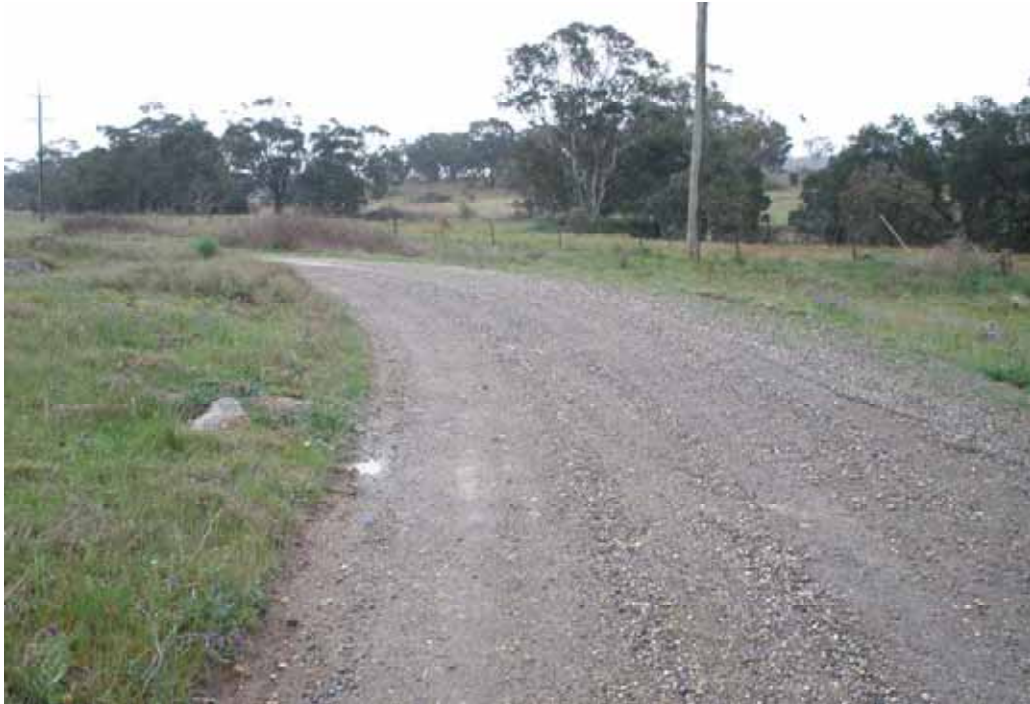
Photo 113 – Stoney Creek Rd (unsealed). Loose aggregate and depressioning along wheel paths.
