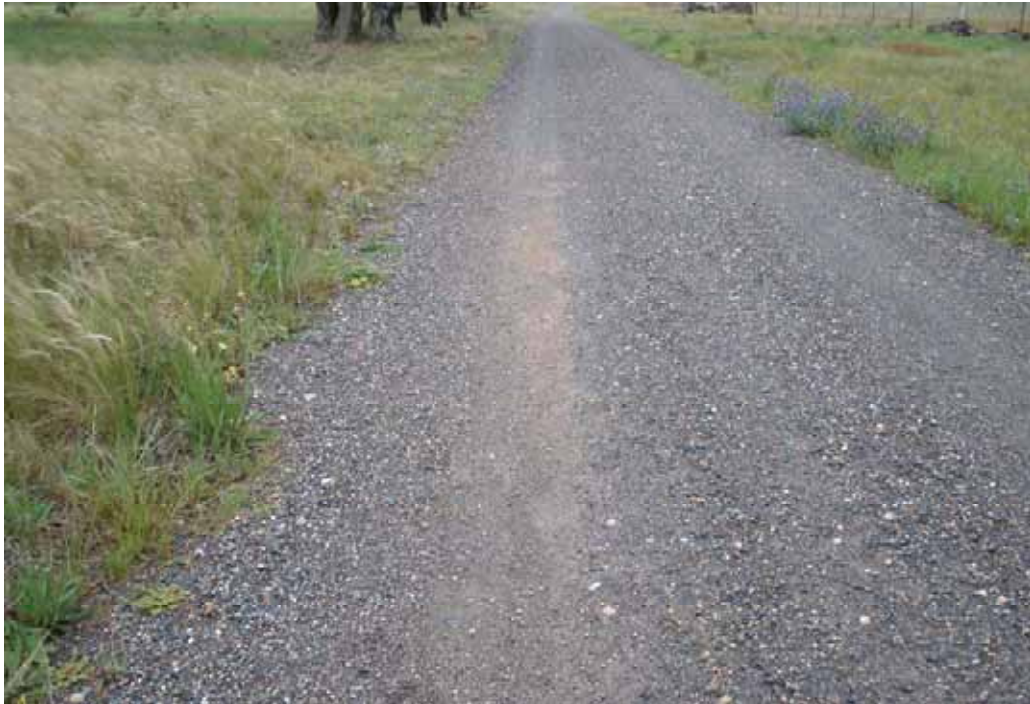
Photo 107 – Stoney Creek Rd (unsealed). Section of minimal gravel southern wheel path.
