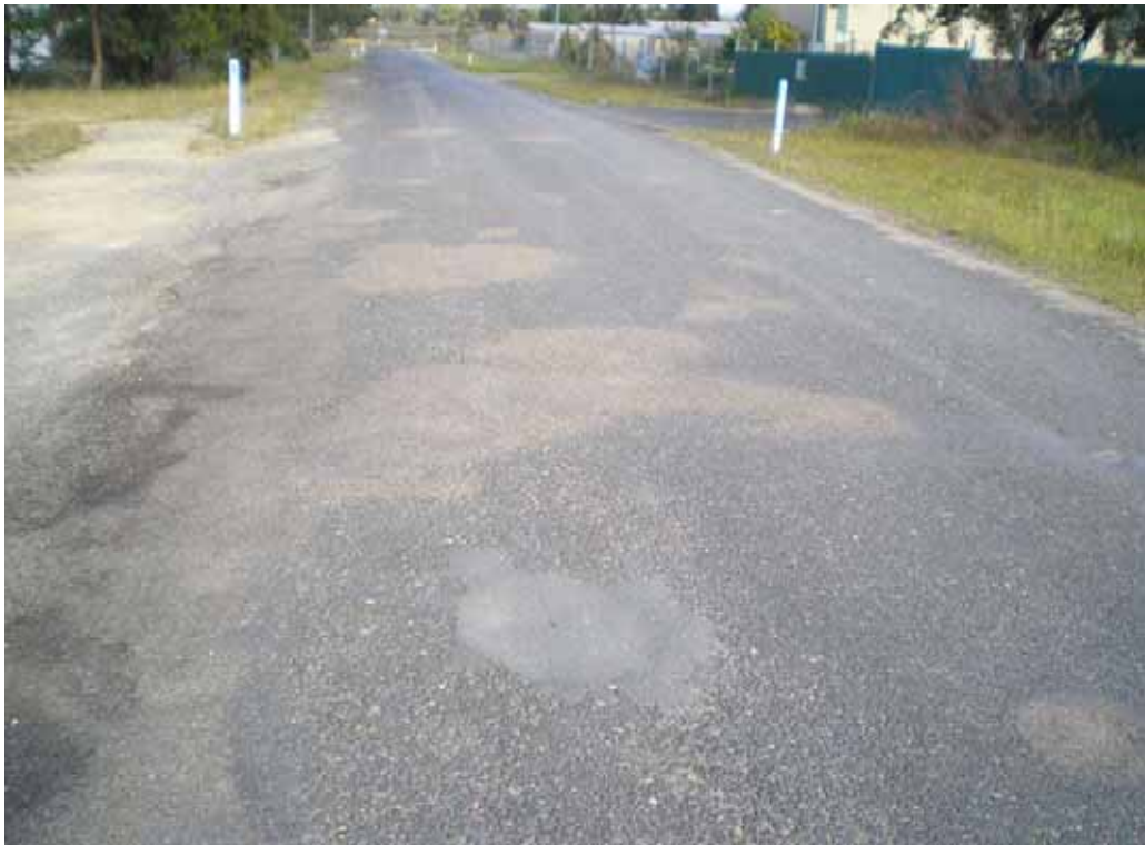
PHOTO 46: Repaired sections/potholes
